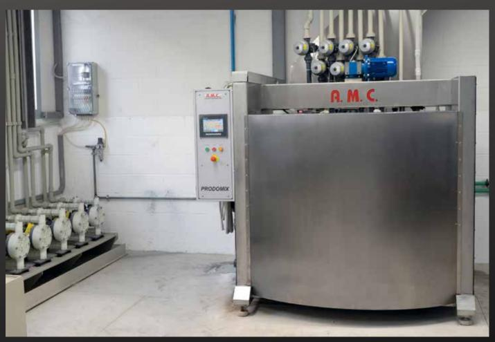
VISTA DI UN IMPIANTO DI PRODOMIX DA 1000LT CON SERIE DI POMPE PNEUMATICHE PER LINEE PRODOTTO VIEW OF A 1000LT PRODOMIX SYSTEM WITH A SEVERAL OF PNEUMATIC PUMPS FOR CHEMICALS LINES
